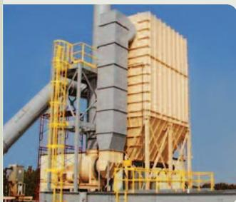
loading felt media. Surface loading allows ProPulse pleated bag filters to capture finer particulate more effectively, along with offering superior release characteristics during pulse-cleaning cycles.
